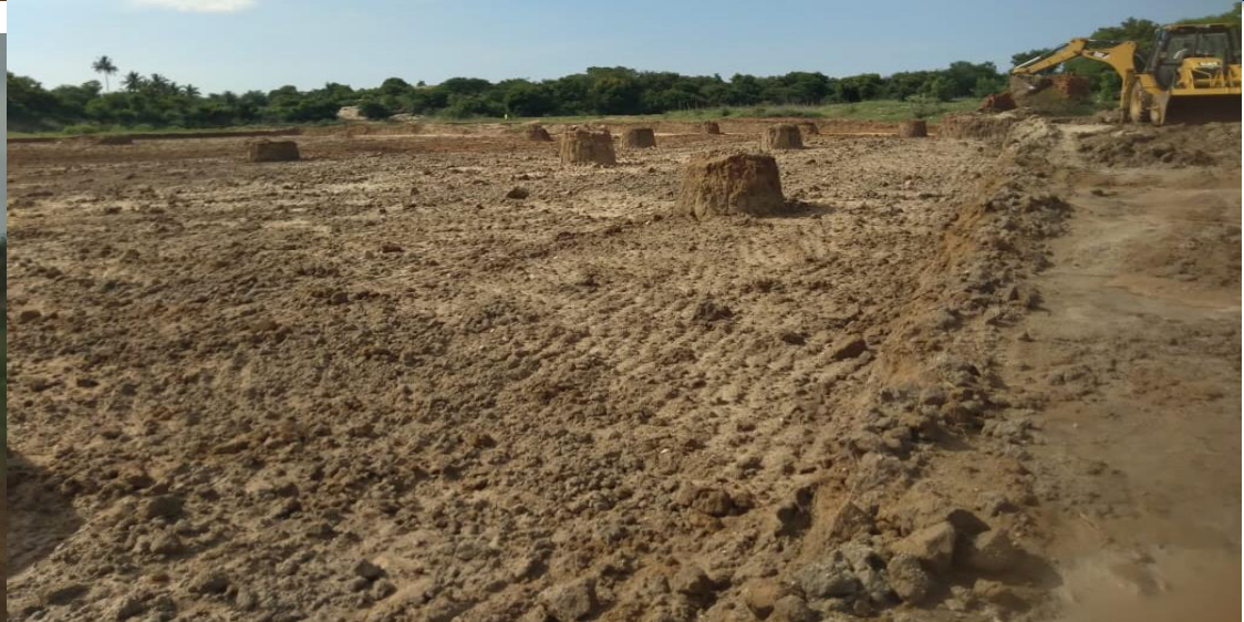
12195 CuM silt complete excavated as goal in Doddathammanahallikere, Mulbagal Tq.
